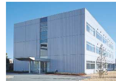
①社屋外観 Front view of main building
