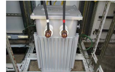
Renewal of substation facilities (Hosoe Factory)
