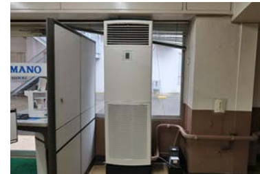
Renewed air conditioners (Head office)
