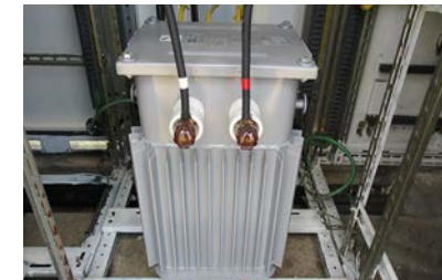
Renewal of substation facilities (Hosoe Factory)
