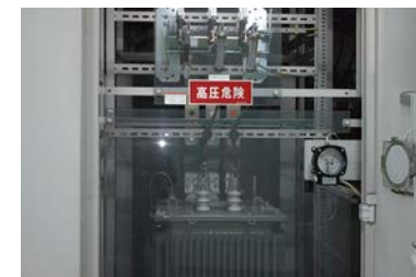
Replaced aging transformers to improve the efficiency of power supply (Hosoe Factory)
