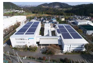
Shifting to self-consumption solar power generation (Sagami Factory)
