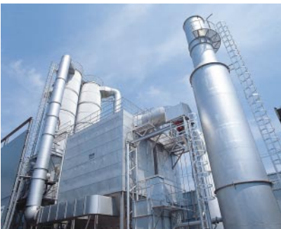
"High-temperature Hazardous Gas Removal System" receives substantial attention as a way to resolve the dioxin problem.
